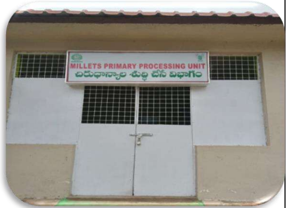
Primary Processing unit
